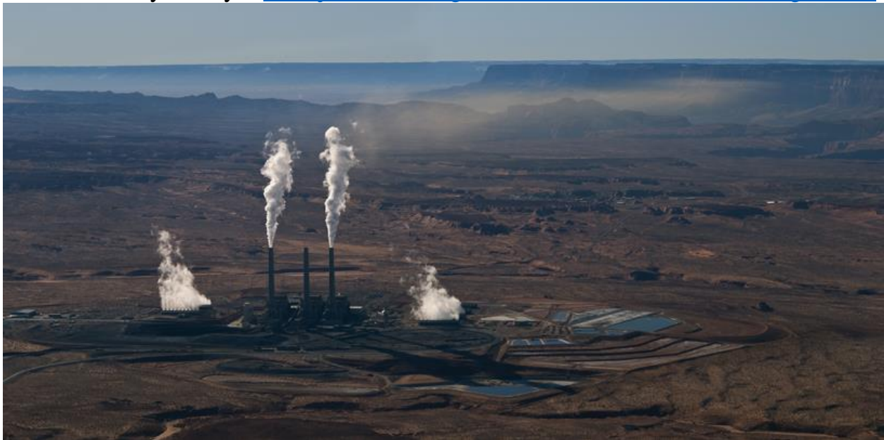
The Navajo Generating Station, one of several coal-fired power plants on or near Navajo territory. Photo by Ted Grussing
